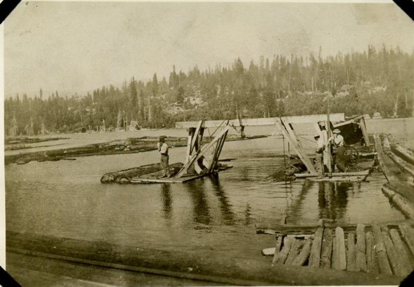
Raising sinkers on Shaver Lake - 1898 - (Photo #44)
